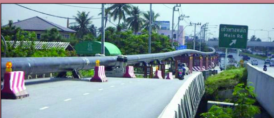
76cm (30") Gas Pipeline – Bangkok, Thailand
