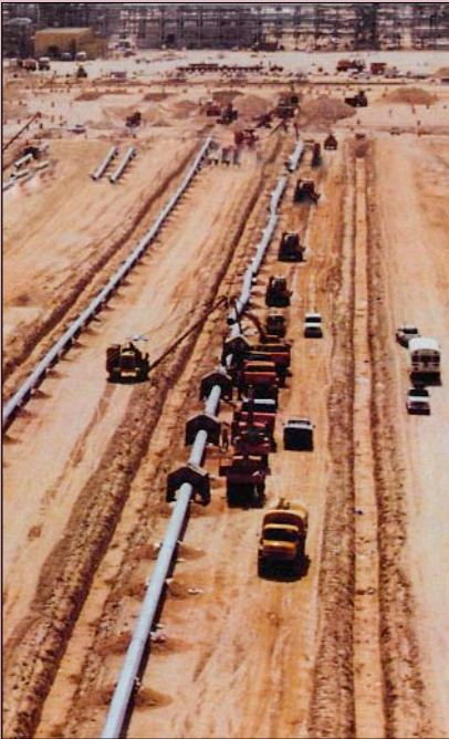
76cm (30") Gas Pipeline – Haradh Project, Saudi Arabia
