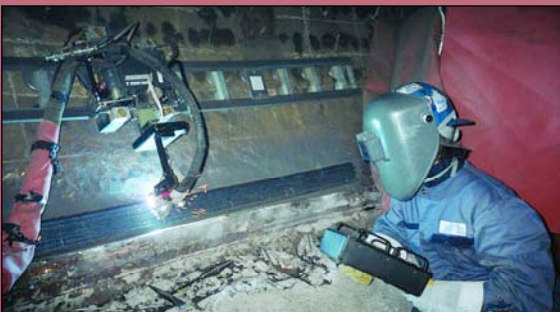
15.2m (50') Diameter ID Weld Build-up – Refinery, Canada
