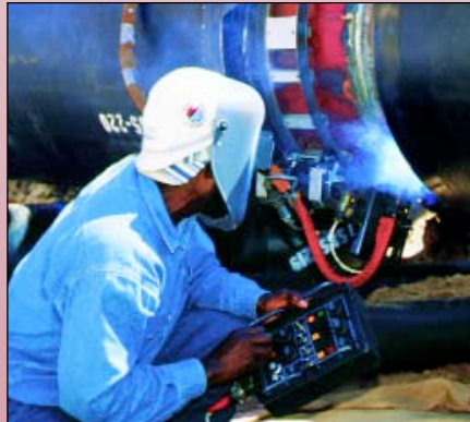
Welding Steam Line – Slattery Project, NYC
